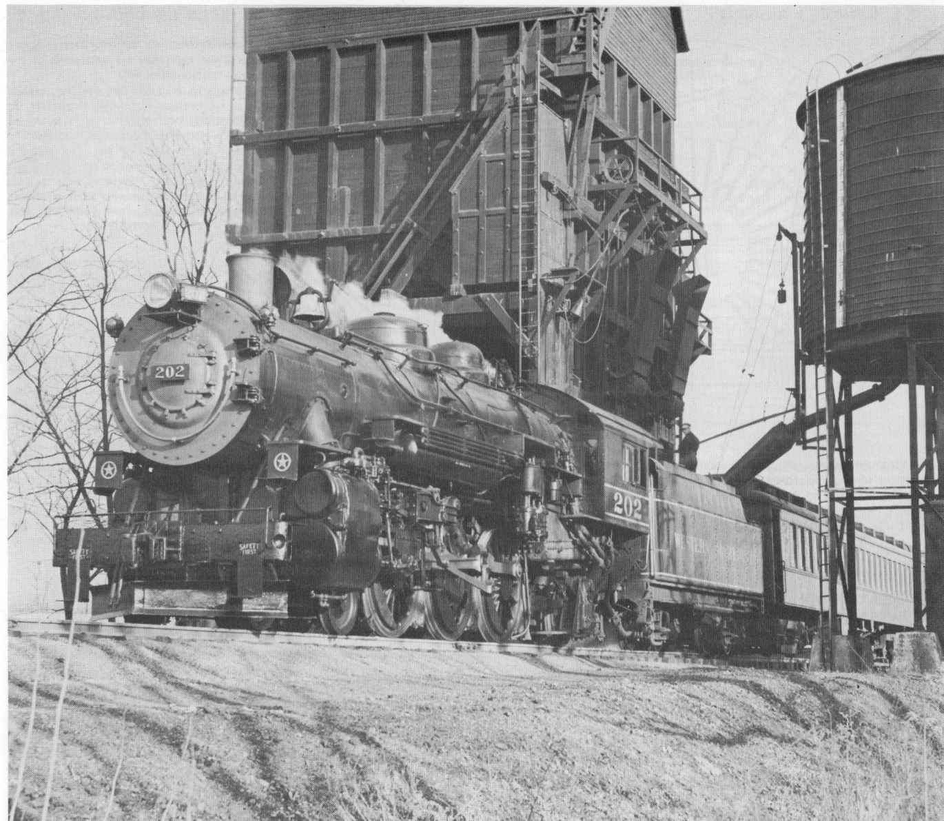
Fig. 4-7. This Western Maryland passenger train stops for water right on the main line. It passed up the coal dock only because it has been converted to burn oil to meet a Baltimore antismoke ordinance. Freight hogs frequently replenished their fuel supply
