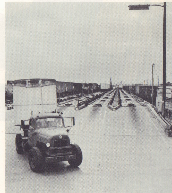
Fig. 1-5B. PRR's "TrucTrain" tracks have lighted walks between them to facilitate loading at night, when most loading is done.
