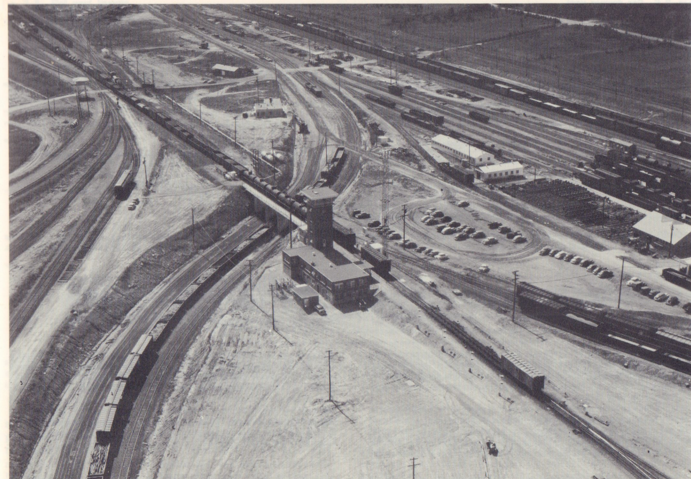
Fig. 2-5. Cars rolling down the hump of the Southern Ry.'s modern Ernest Norris Yard, Birmingham, Ala., pass a glassed-in inspection pit and an automatic journal oiler before crossing the overpass. The track arrangement takes advantage of the hump's elevation to provide uninterrupted access of both rail and automobile traffic from one side of the yard to the other. The first
