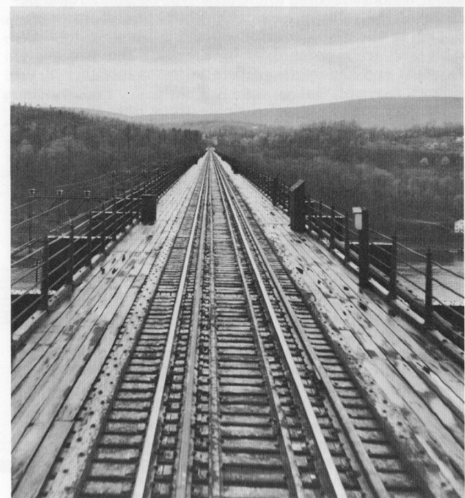
Fig. 3-10. Six-rail track? No — gantlet track plus two guard rails (without tie plates) in the center. The New Haven RR. gantleted the formerly double-track line over Poughkeepsie Bridge to keep the weight of locomotives centered so that the structure, dating from the 1880 era, could handle modern 2-10-2 motive power without being rebuilt.
