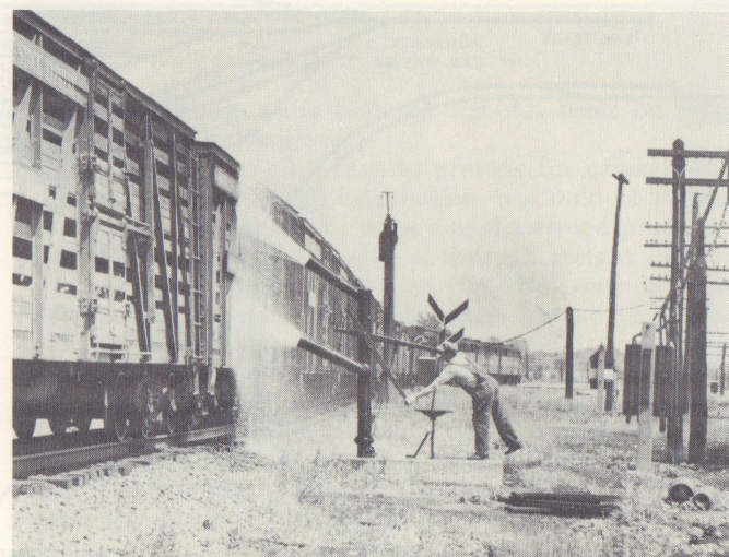
Fig. 4-11. Hog-flushing penstocks on the New York Central cool off double-deck loads of porkers as they pass through on a hot day. Hogs (the only exception to the 28-hour rule) can be rested and fed in the cars if they have room to lie down.
