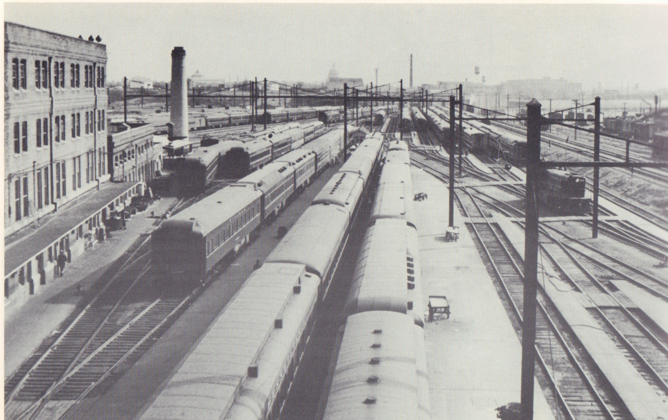
Fig. 4-10. Coach yards serving Washington Union Station are located within the wye track used to turn entire passenger train consists. Note narrow concrete platforms located to serve both sides of cars on body tracks in subyards into which huge yard is divided. Subyard ladder tracks lead directly to lead tracks ex-
