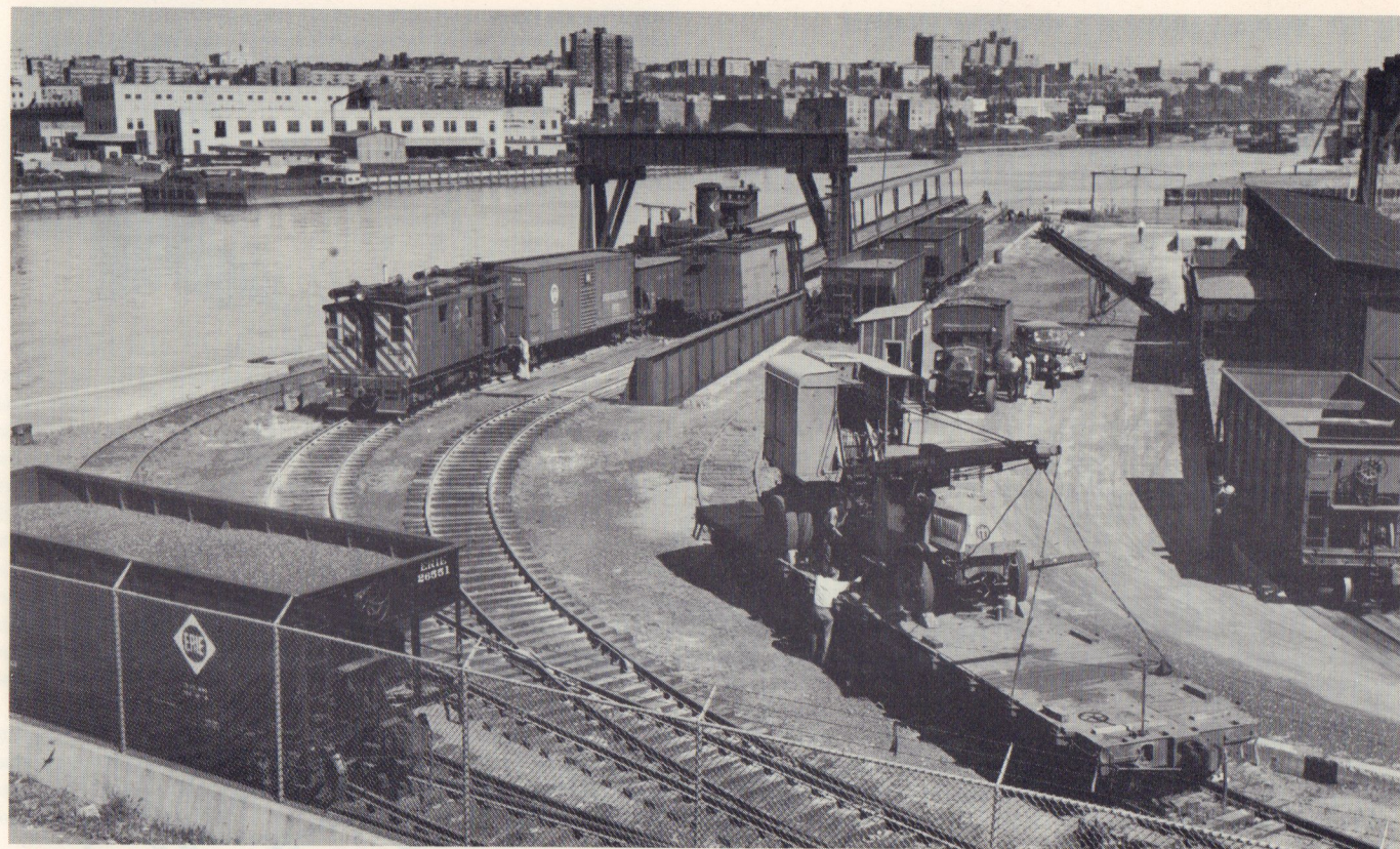
Fig. 7-4. This is a capsule edition of a big railroad—the Erie RR. car-float terminal on the Harlem River in New York City. Cars brought by water from the Erie's huge Jersey City terminal are wrestled around the sharp curves of this vest-pocket yard by a single diesel that serves team tracks and industry sidings
