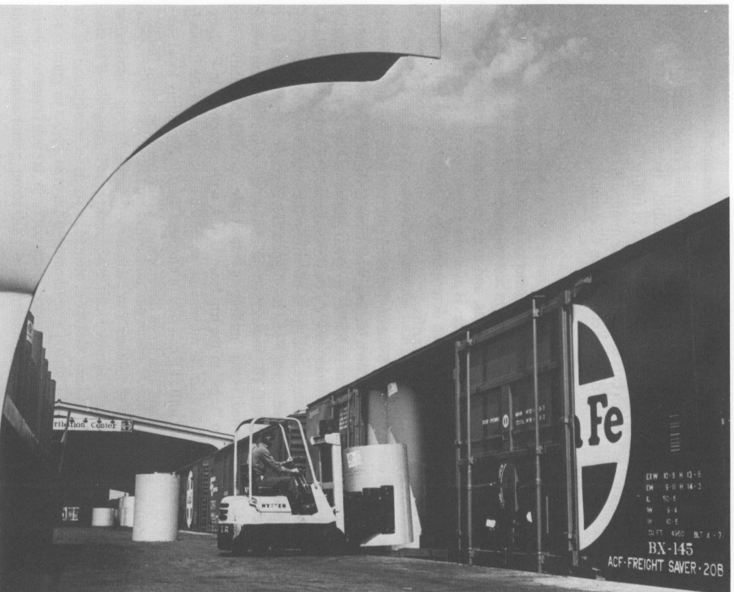
Fig. 8-1. Team-Track Loading Facility
