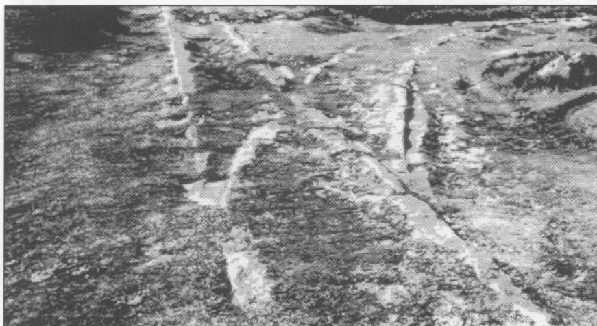
Fig. 1-3. Photo shows the remains of a turnout on an early 19th century predecessor of today's railroad – a 10-mile tramway transporting dressed granite from quarries on Dartmoor in Devon, England, down to a canal leading to the sea. Guiding surface on rows of separate granite blocks forming the “rails” allowed 12 four-wheel wagons to be assembled into trains to roll their loads down to sea level by gravity. Empty trains were hauled back up to the quarries by teams of up to 19 horses. The gauge of the stone faces guiding the 3-inch-wide plain treads of the wagon wheels was 4 ft 3 in. Turnouts, such as this with a single stone “switch point” pivoted on an iron pin, allowed trains to meet each other and to be guided into spurs serving different quarries.
