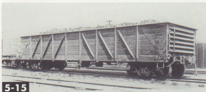
5-15 Thousands of 50-ton USRA composite gondolas were built, featuring a steel underframe, ends, and bracing, with wood sides. David P. Morgan Library collection
