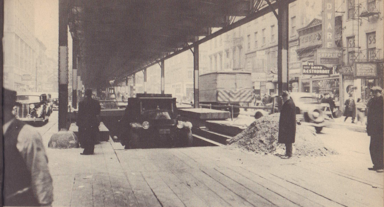
The truck is getting its load of dirt (above). Here excavation is done directly by power shovel, which digs into the heading, swings around with its beak full of earth, and dumps it into the truck. Below—A loaded truck just emerging from the ramp.
