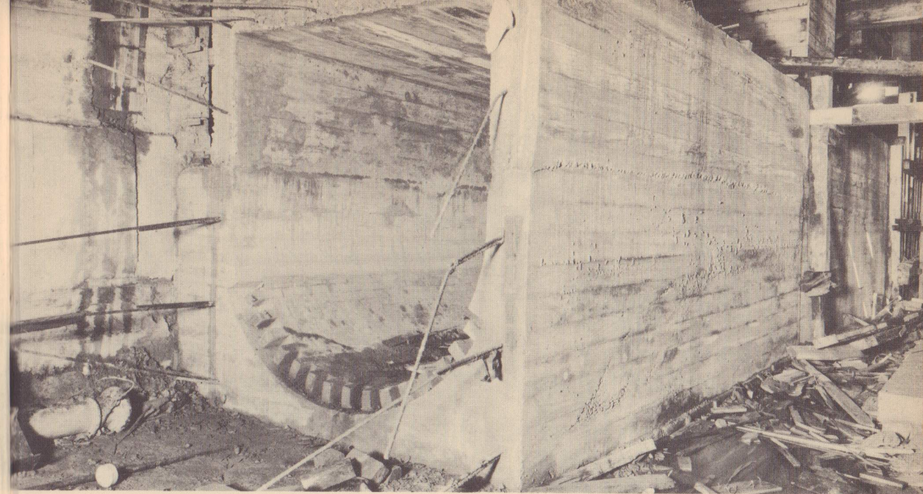
An enormous concrete sewer being built according to specifications of the Sewer Department of the City, by the construction contractor. Sometimes they come even larger! Below—Concreted steel (right), naked steel (left) and the duct banks being laid along the side of the structure.
