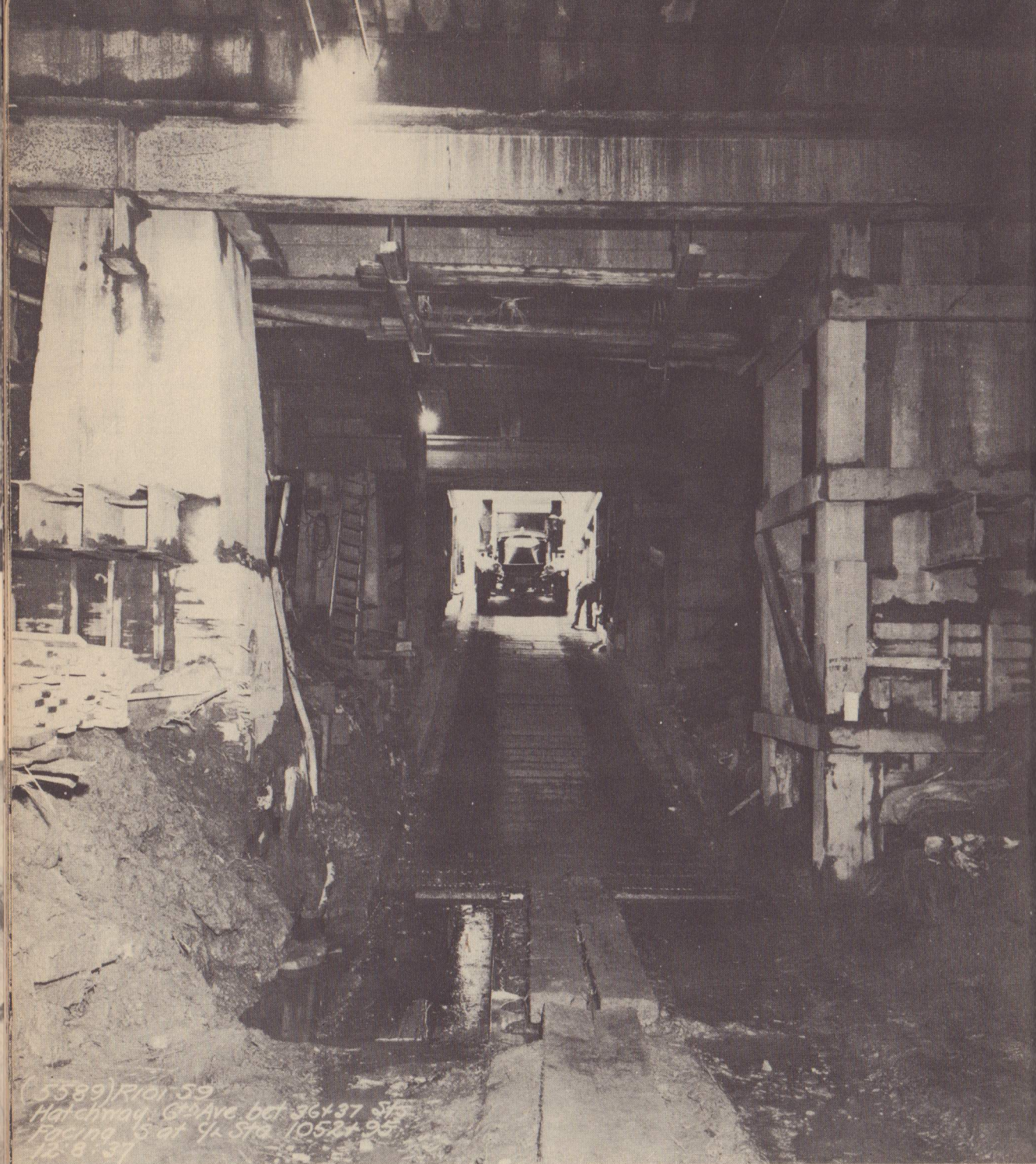
Coming down a ramp. The truck must come down in low gear, very slowly, for the grade is extremely steep.
