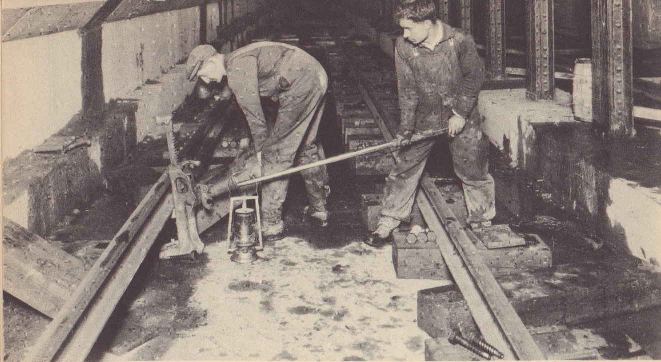
The short ties, always used with type II track, being inserted under the rails. The rails have been loosely bolted together along the length of the subway, and the ties are put in place by means of a hand jack, which lifts the rail so that the tie can be pushed under it. Below—The ties are all in place, and the rails are being spiked to them, with power drivers. Note the air compressor machine. It furnishes the power to the spike drivers.
