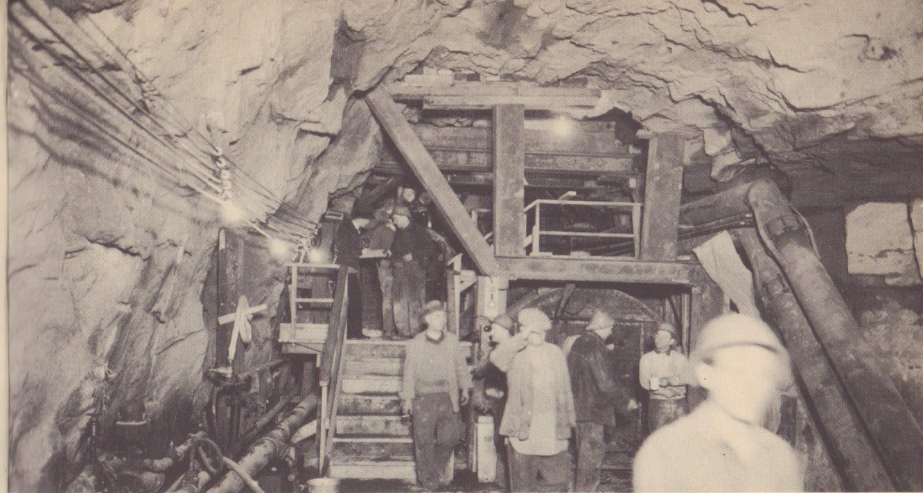
After working for the two or three hours their shift lasts, the men (above) are coming out of the man-lock. Now they'll go off and drink lots of hot coffee and rest up for an hour or so before going on for another two or three hour shift. Below, an engine preparing to pull a loaded car out of the muck-lock. (Bottom photo, courtesy of Spencer, White and Prentis.)
