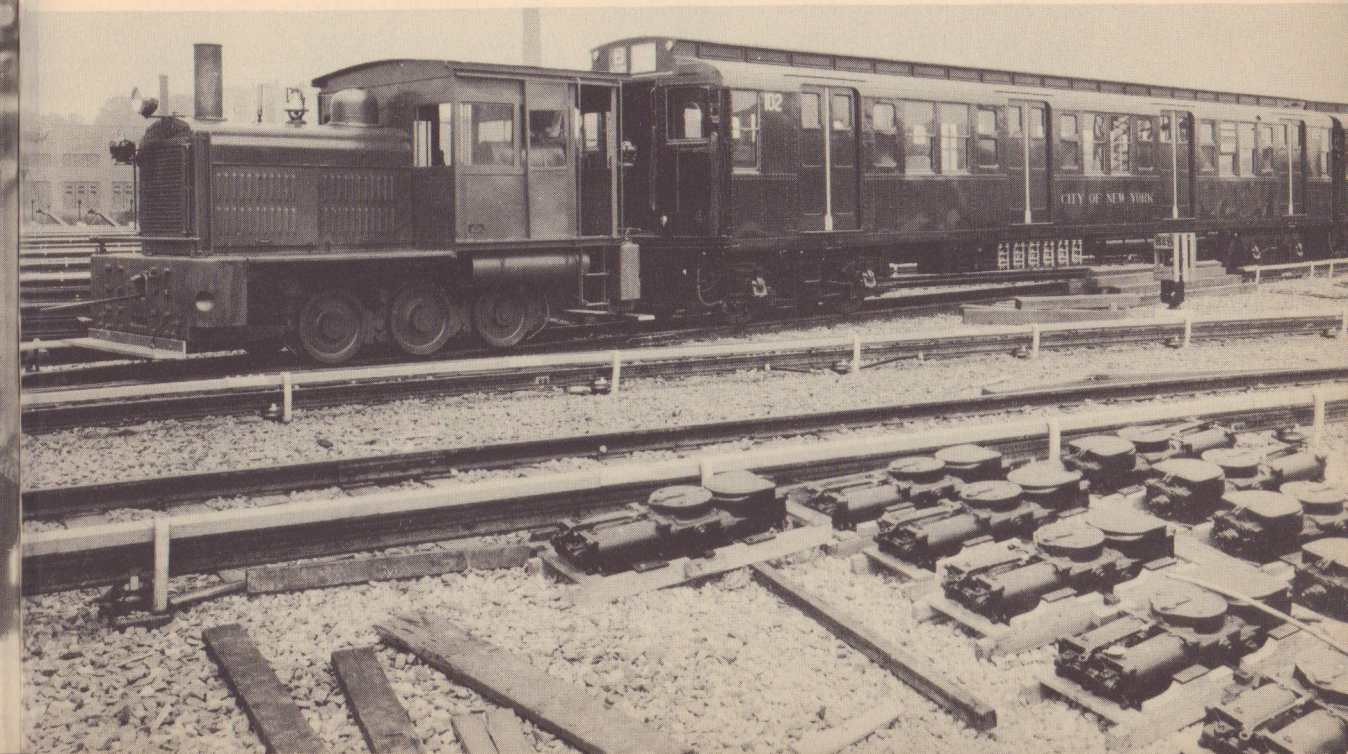
A bird's-eye view of the subway yards. Below—A yard engine hauling some new subway cars. Note the row of switch mechanisms in the foreground. They are still crated, you will note, and are waiting to be installed down in the subway as soon as they are needed.
