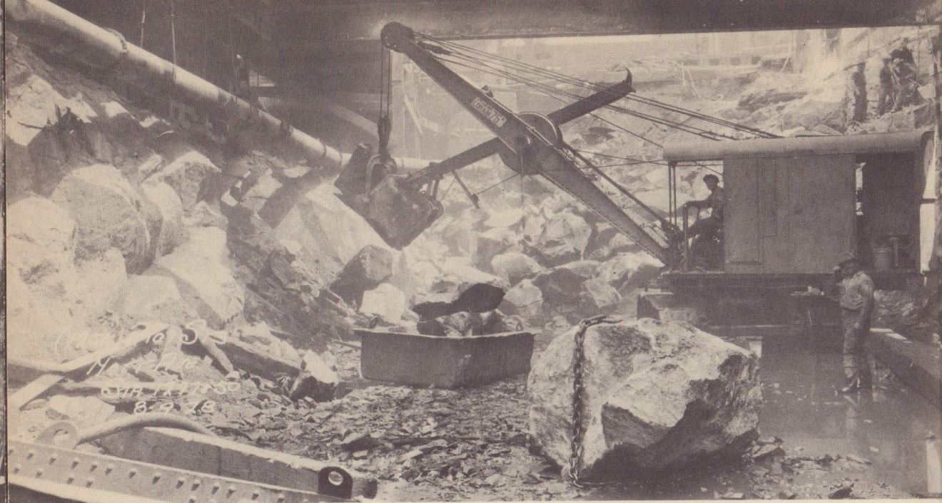
Two types of excavation buckets. Above—A power shovel is piling rock into a "tip-over," which an overhead crane will pull up when full. Note the chain around the big boulder. It will be hoisted by the chain. In the bottom picture, a type of battleship muck bucket is dumping its load into a waiting truck. (Bottom photo, courtesy of Spencer, White and Prentis.)
