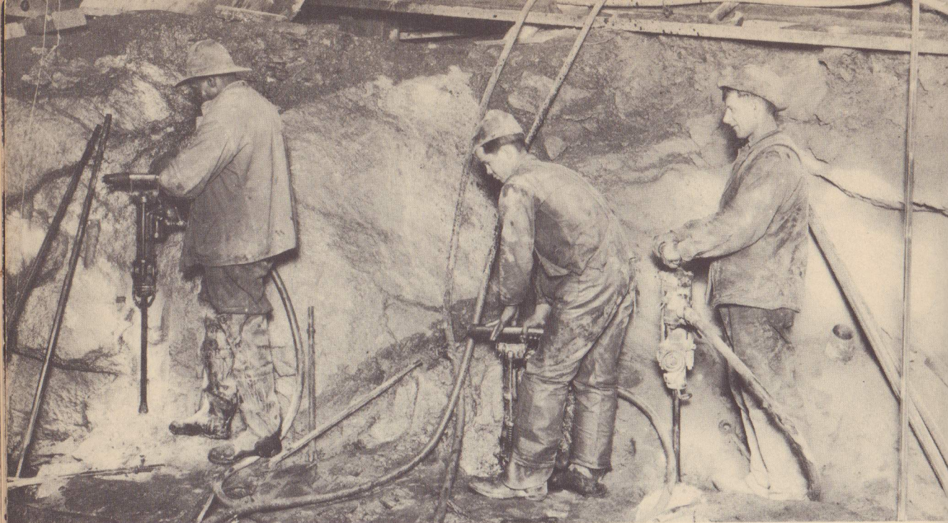
The drillers in the picture above are working with short drilling arms, and are putting down dynamite holes right up against the heading. The next blast may knock out several feet of the rock. Below, a blast has been set off, and the workmen are clearing up after it, pushing pieces of broken rock down to the bottom.
