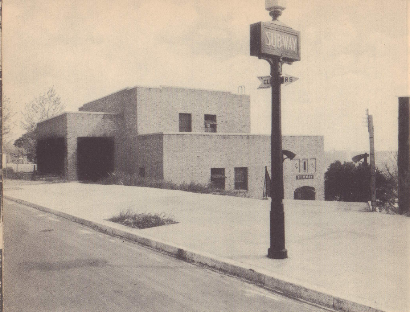
Here is a different kind of subway station in New York. It houses the mechanism for several elevators, which take passengers more than 75 feet down to the level of the subway! The station is up at Washington Heights, Manhattan, where the trains run clear under a sizable hill.
