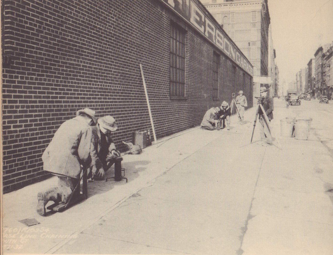
"Chaining"—the technical name for the measuring of the space between stations with a special metal tape measure. The surveyors must measure the distances with absolute accuracy.
