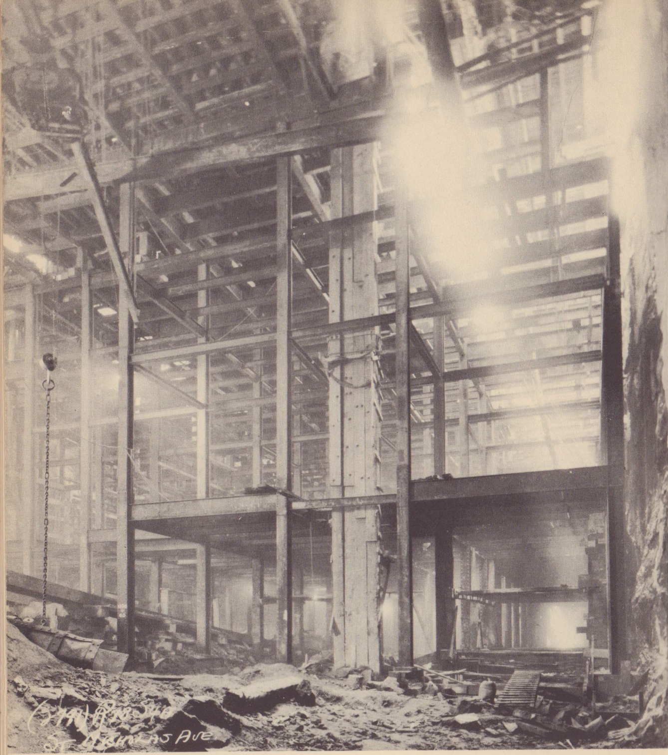
A maze of steel. At this point, there are three levels which you can count in the steel frame. The bottom two will carry tracks; and the third will be the mezzanine of a station.
