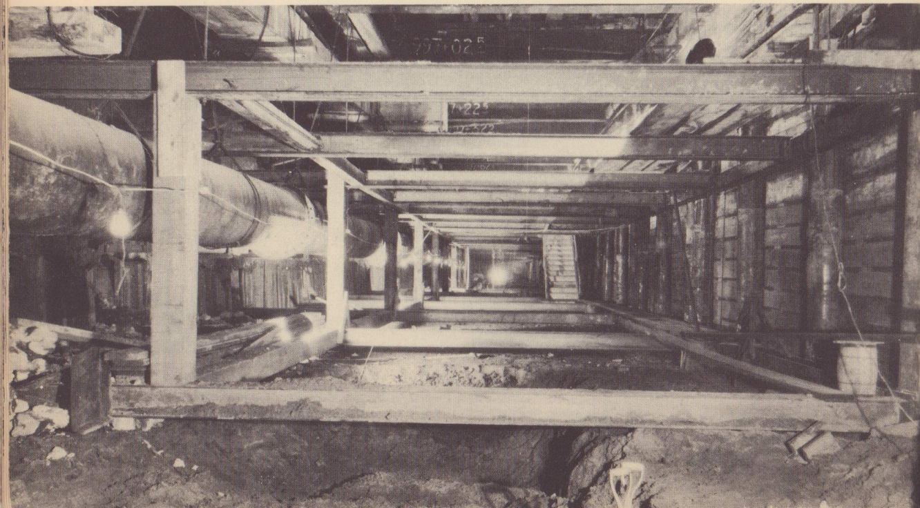
Another view of wood shoring, above. But notice, below, how much clearer the excavation is when steel is used. Sometimes, of course, even more steel has to be put in, but it never is as confused as it is with wood. (Bottom photo, courtesy of Spencer, White and Prentis.)
