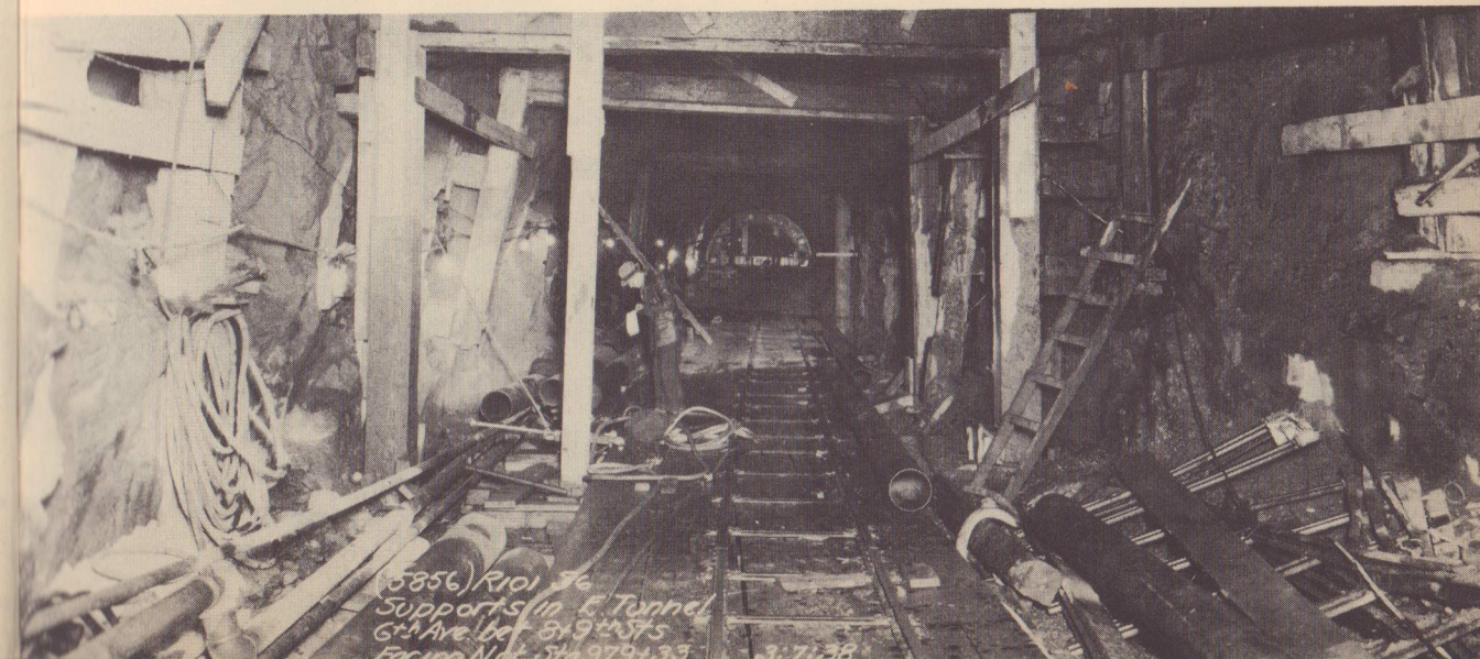
The shield from the rear. The "tail" is the part which sticks out beyond the main part of the structure; and those queer objects placed about two feet apart all around the shield inside the tail are the hydraulic jacks used to push the shield ahead. Below is the way the shield, as assembled, looked from a distance.
