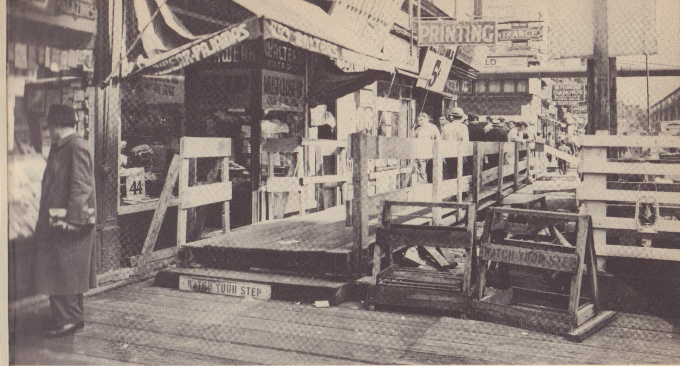
Here is a place (above) where the sidewalk decking is only a narrow bridge. Excavation work is going on where the rest of the sidewalk should be. The strange looking little outhouse in the picture below is actually the entrance to a flight of steps going down to the excavation itself. This is the way the workmen get down to their jobs.
