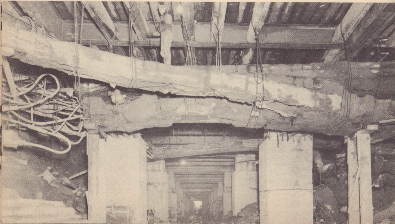
Subsurface structures. Above is a duct-bank which has been broken apart, and each pipe separately cared for. Below—A bank of ducts left intact, and suspended from the decking as it crosses inside the subway structure.
