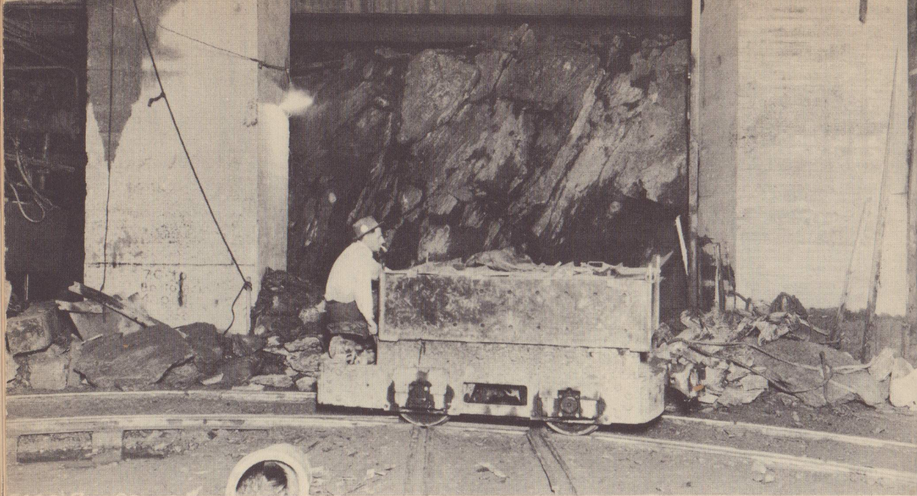
Industrial track. The storage battery engine is above. It goes very quietly, of course, and not very fast. Below, one of the miniature power shovels which have been specially designed for small tunnel work, busy loading rock into a bucket on an industrial-track car.
