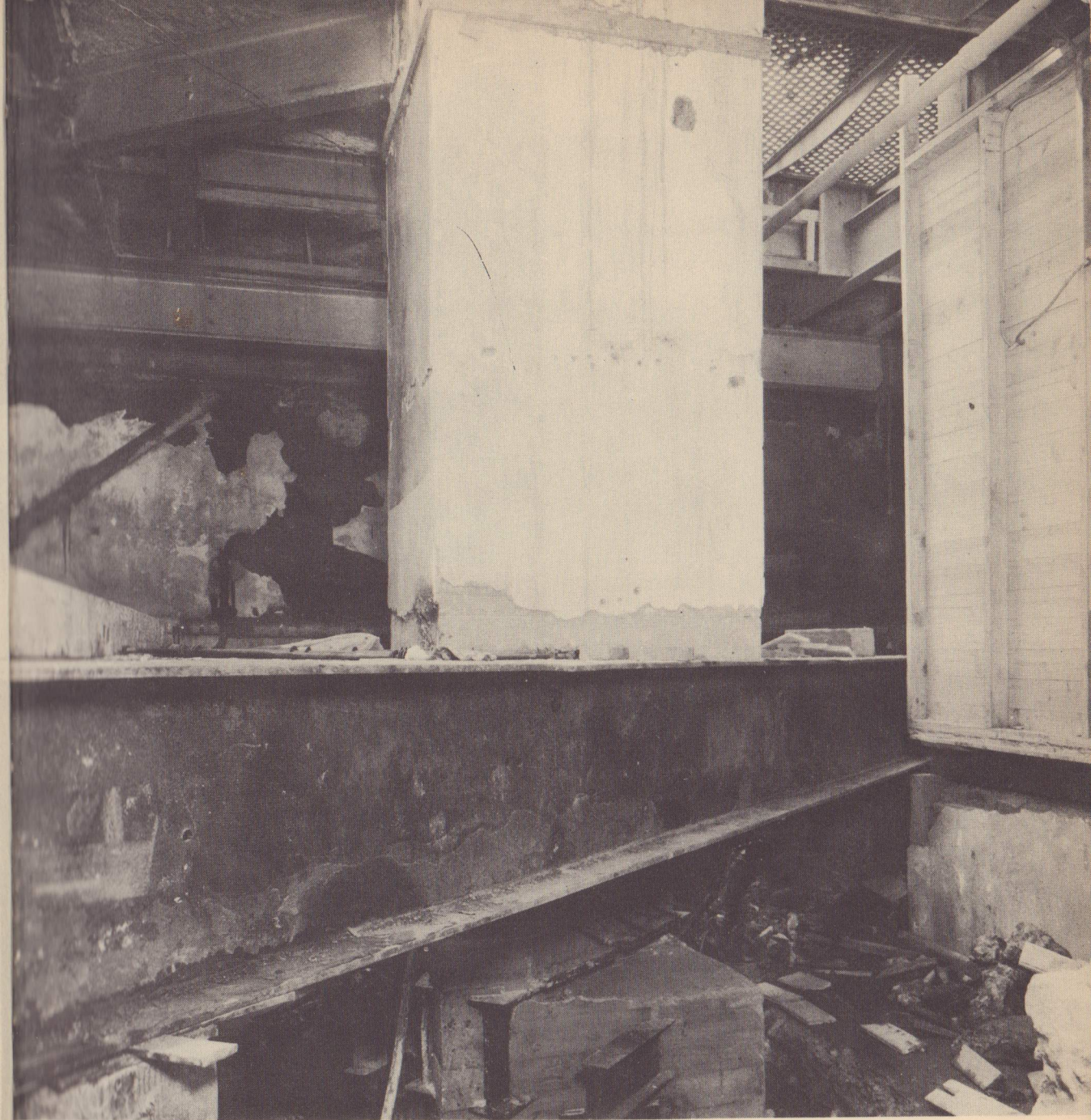
A sidewalk vault has been taken over by the city, so that underpinning of the foundation of the building itself can be done. Note the "sidewalk lights" in the upper right-hand corner (the glass blocks which let light into the vault). To the right is a wooden partition which protects the rest of the basement from the excavation. The great steel beam on which the pillar of the building foundation rests is a type of needle-beam, used when foundations are in the form of pillars, and not continuous walls.
