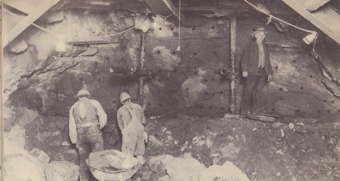
Two types of drilling holes. The heading above is completely riddled with holes, so that the whole area will be blasted loose. The row of holes in the picture below is just enough to break up the particular rock the holes are in. (Bottom photo, courtesy of Spencer, White and Prentis.)
