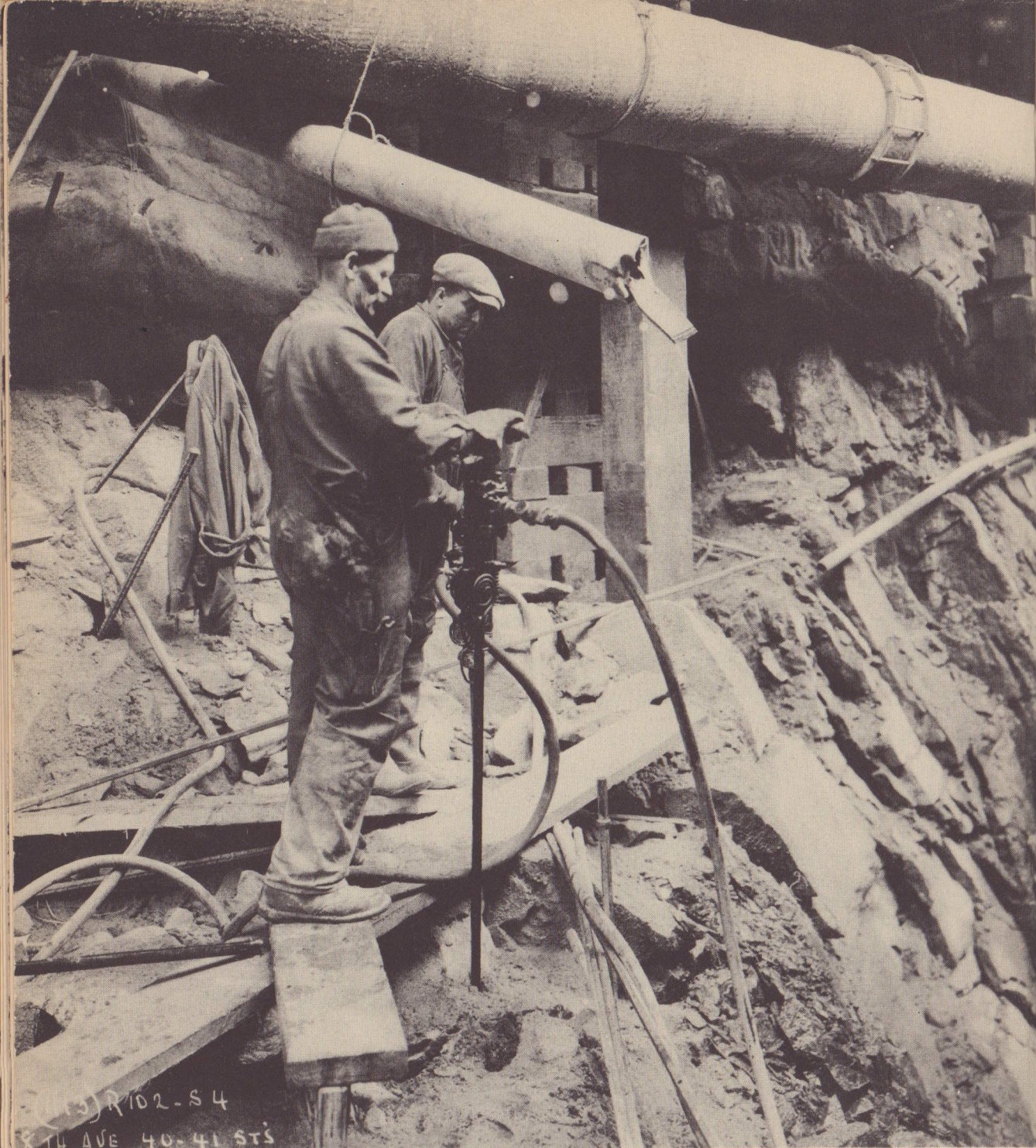
Closeup of a drilling machine. Note how long the drilling arm is. A man has to stand above the surface into which he is drilling, in order to be able to hold the machine upright.
