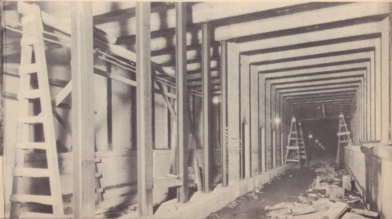
Structural steel going into place in an open cut. Note that concrete is also being poured in this picture. Below—Further steps in construction. You can see in the foreground (left) the naked steel girders—and in the background, the same row of girders encased in concrete to form the collision wall.
