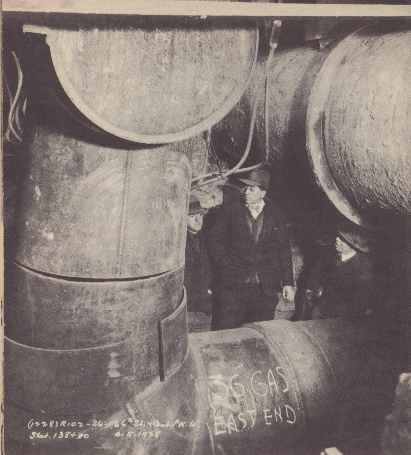
Three men and some pipes! A new gas main is being installed.
