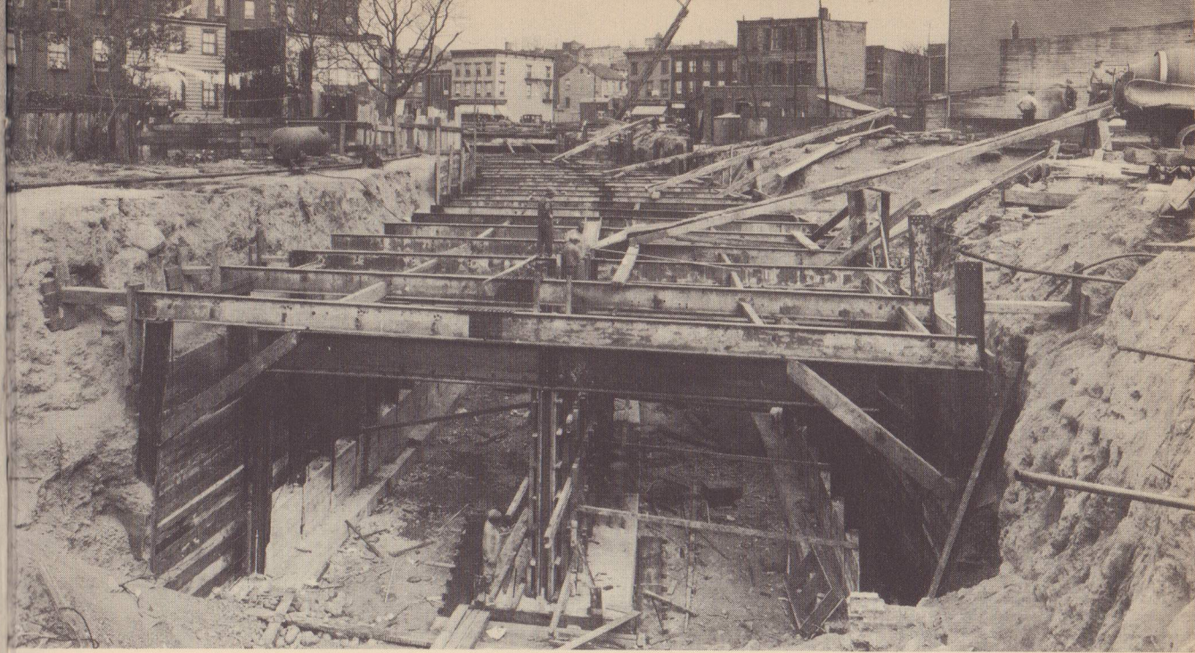
Structural steel going into place in an open cut. Note that concrete is also being poured in this picture. Below—Further steps in construction. You can see in the foreground (left) the naked steel girders—and in the background, the same row of girders encased in concrete to form the collision wall.
