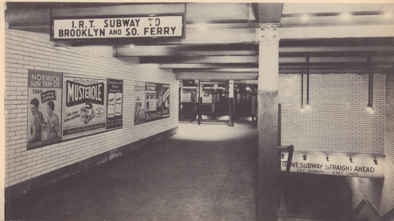
A station entrance. It is built into a regular building alongside stores. Entrances used to be from sidewalk stairways, but now they are through such buildings as in the picture above, whenever possible, so that the sidewalk can be kept clear of obstruction. Below is a view of a finished station, showing the advertising plaques in the walls.
