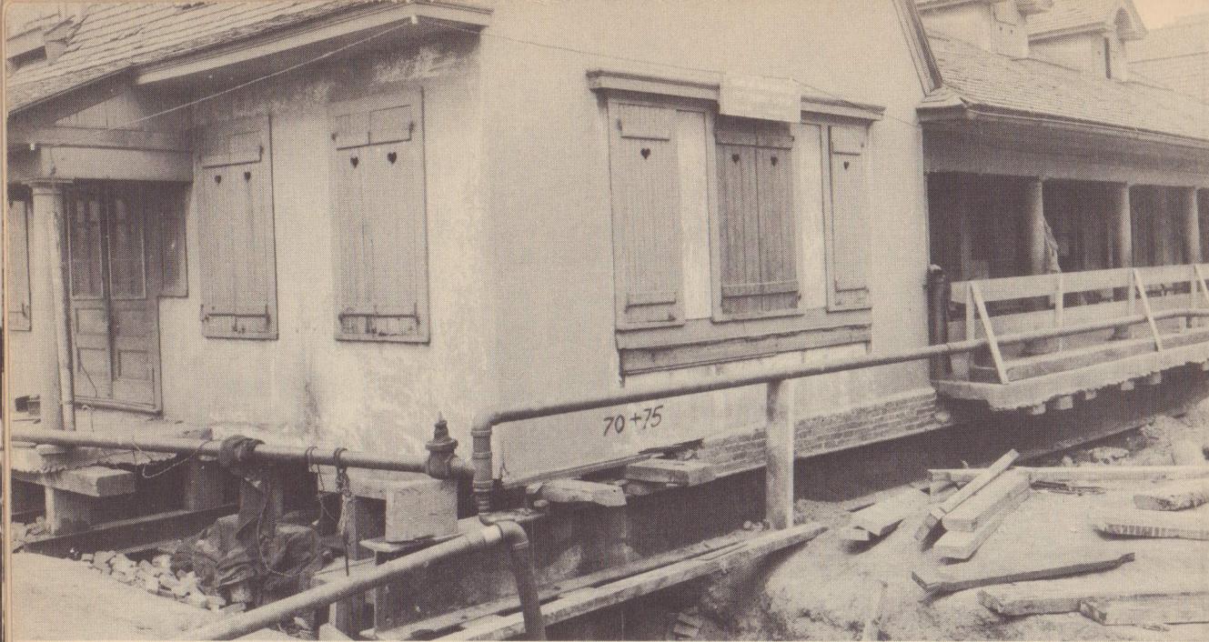
The two types of underpinning. Above, a "grid-beam," supporting a small frame building. The foundation has been cut away, and the building rests on the steel beam. The "needle beam" below is holding up a section of extremely heavy wall, so heavy indeed that there are two needle beams in the same hole.
