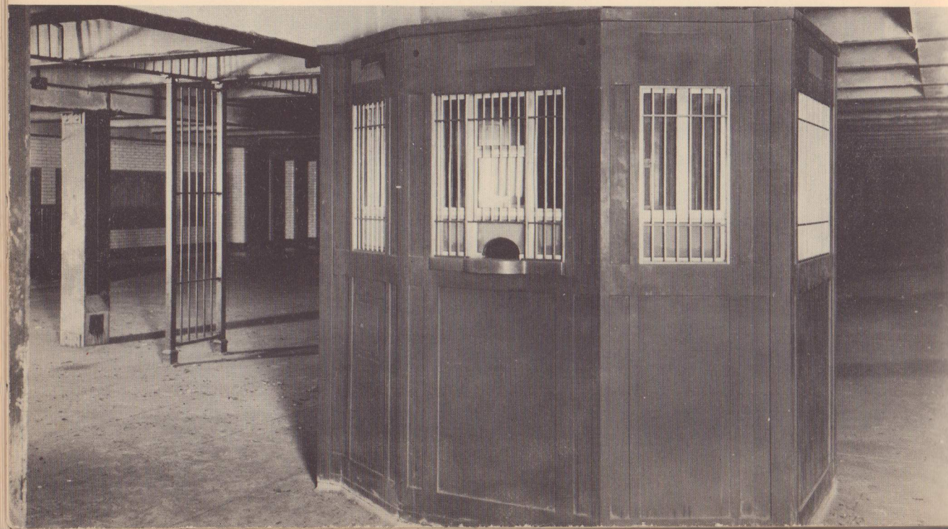
Station finish. A row of automatic turnstiles, operated by a nickel in the slot, is shown above, together with a specially built-in change booth, just beyond the turnstiles. That type of change booth is no longer used on the new subways. The one shown in the picture below is standard equipment nowadays.
