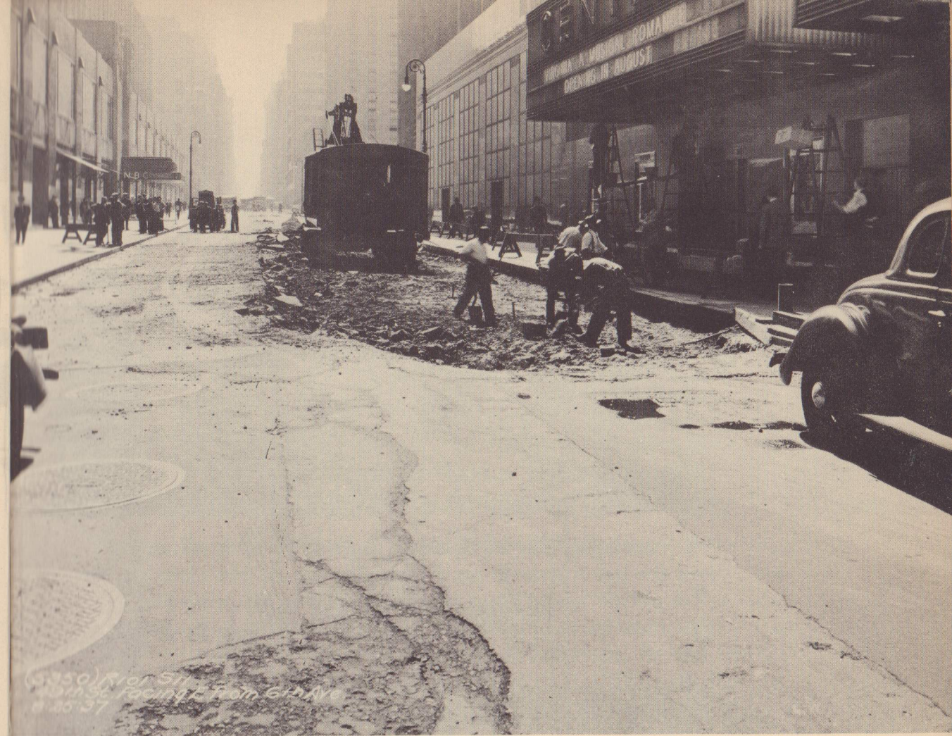
Breaking up the street surface, preparatory to excavation. Here the shovel is picking up the large hunks of asphalt and concrete previously broken up by workers with their air-power drills.
