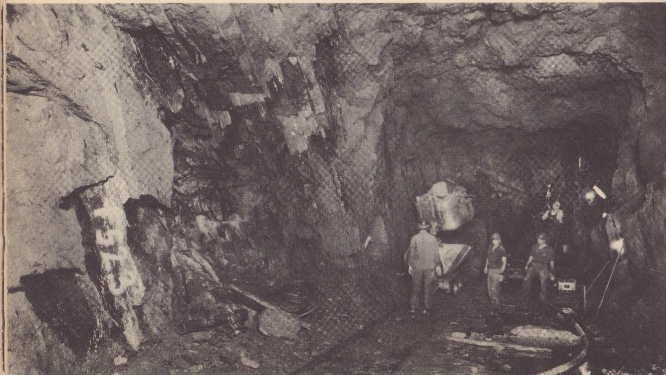
Industrial track. The storage battery engine is above. It goes very quietly, of course, and not very fast. Below, one of the miniature power shovels which have been specially designed for small tunnel work, busy loading rock into a bucket on an industrial-track car.
