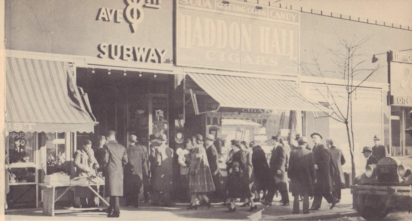
A station entrance. It is built into a regular building alongside stores. Entrances used to be from sidewalk stairways, but now they are through such buildings as in the picture above, whenever possible, so that the sidewalk can be kept clear of obstruction. Below is a view of a finished station, showing the advertising plaques in the walls.
