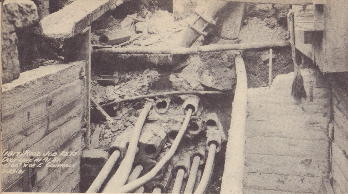
Subsurface structures. Above is a duct-bank which has been broken apart, and each pipe separately cared for. Below—A bank of ducts left intact, and suspended from the decking as it crosses inside the subway structure.
