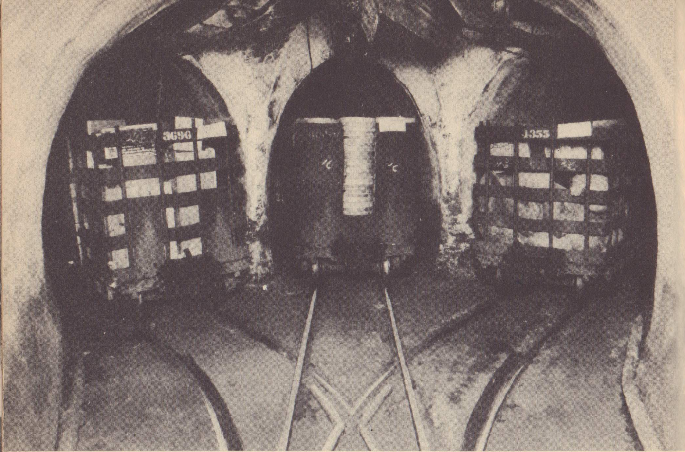
Chicago's queer freight subway. The picture above shows how small the tunnels are, barely big enough to let the cars through. Below, the "X" marks the place down which the refuse which resulted from the tearing down of an old building on this site is dumped. Underground it is carted off to disposal points far away. (Courtesy of the Chicago Tunnel Co.)
