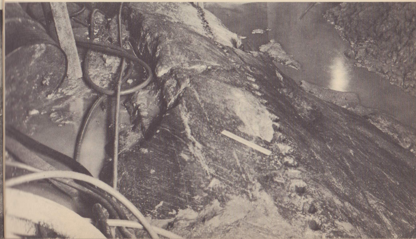
Two types of drilling holes. The heading above is completely riddled with holes, so that the whole area will be blasted loose. The row of holes in the picture below is just enough to break up the particular rock the holes are in. (Bottom photo, courtesy of Spencer, White and Prentis.)
