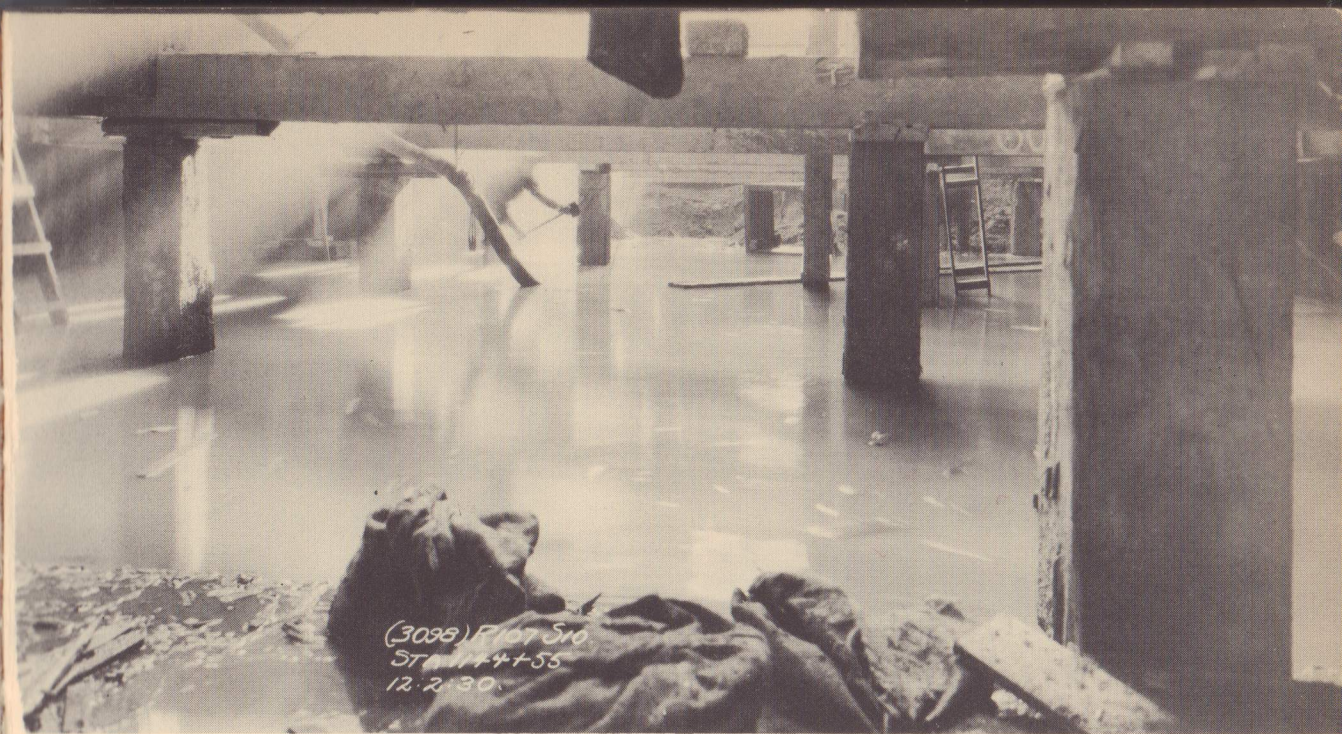
Water in a subway cut. Floods like that do not often occur; but to keep such things from happening at all, the drainage ditch (below) is usually dug. Then the water runs off, and people can work with less discomfort.
