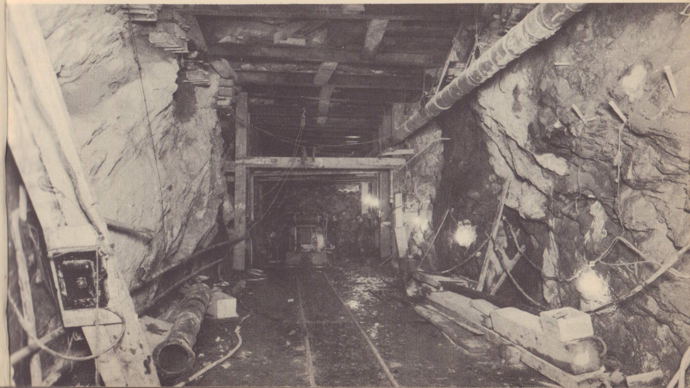
Straight rock tunneling, without even much water to bother you. Here (above) the tunnel is going to be so high and wide that the men can work on two levels—one on the ground, and one on a platform. Below—A much smaller tunnel. The rock is badly faulted, and temporary overhead shoring is needed near the heading to protect the workers from falling boulders, and also from collapse of the side walls.
