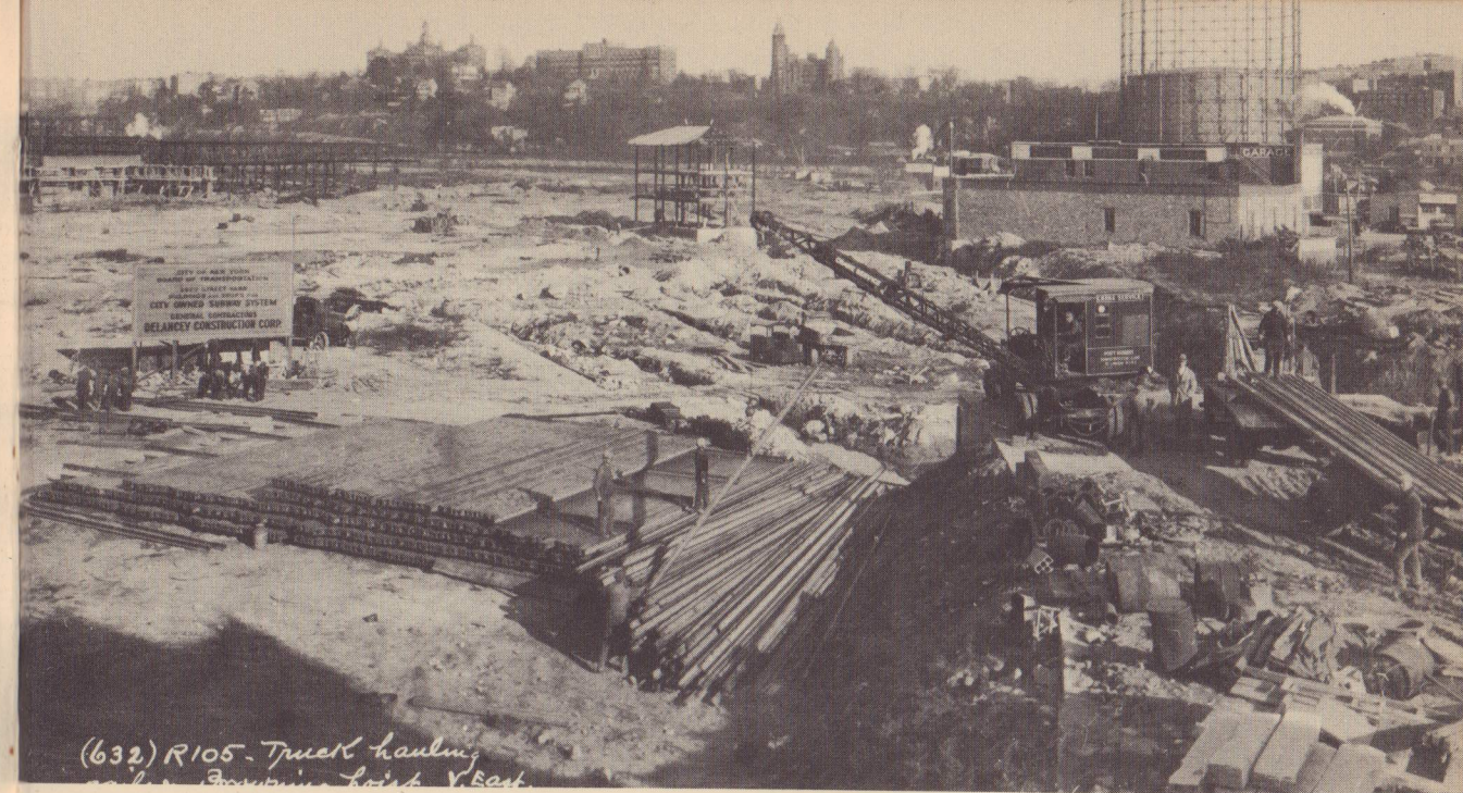
(632) R105. Truck hauling Piles of track stored and waiting to be hauled down into the new subway and to be put in place. The crane lifts one rail at a time and places it on the waiting truck at the right of the picture. The same truck, in the picture below, is shown down in the subway with its load of rails being taken off and placed along the side of the structure.
