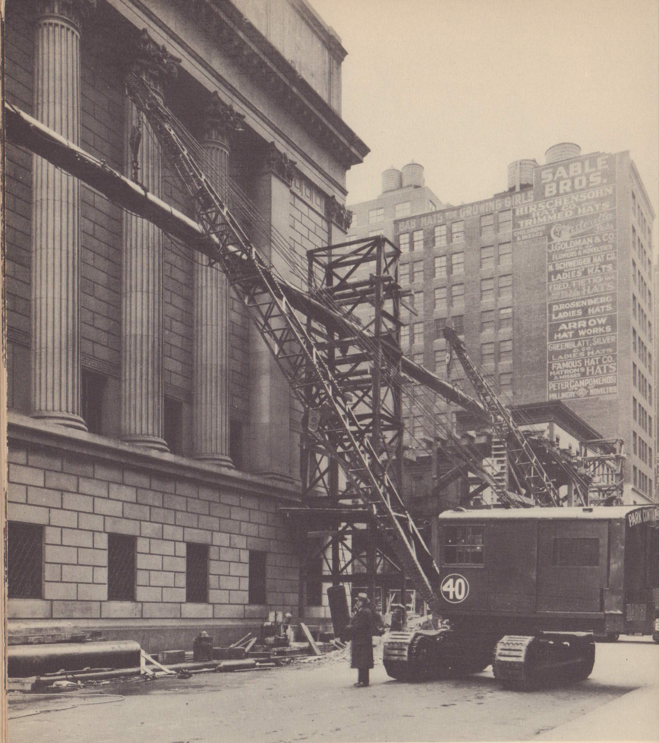
Lifting an overhead bypass pipe into place. The crane holds it up while men (not visible in the picture) make it secure to further sections of the pipe.
