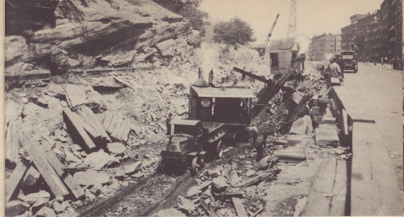
Excavation in open cut. No decking is needed. Above, a very wide street, with digging going on along half of it, without any temporary roadway. Below—Excavation across a vacant area.
