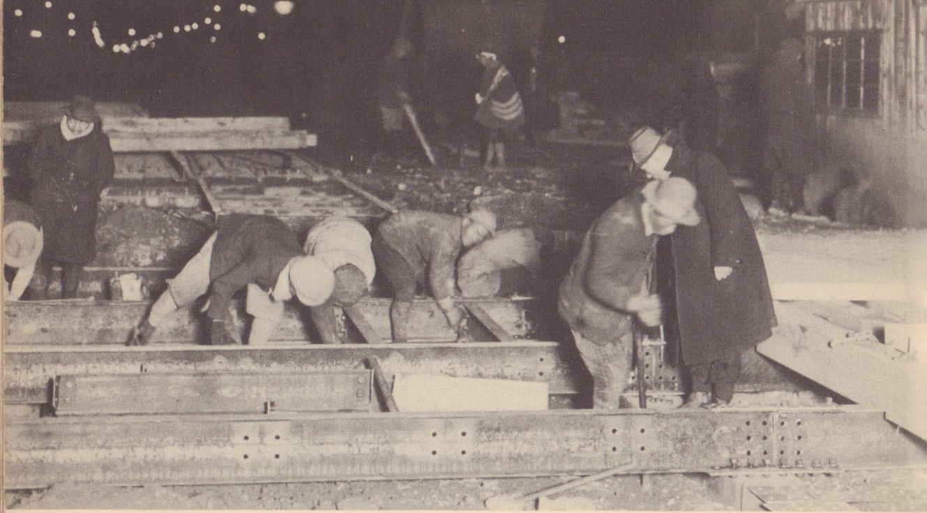
Working at night on the Tokio subway. Here they are building decking, under which excavation will go on. They shut the traffic off entirely at night while the work is going on. (Courtesy of "The Engineering News Record.") Below—The inside of a Tokio subway station. Note the modernistic lighting in the ceiling. (Courtesy of the Japanese Consulate.)
