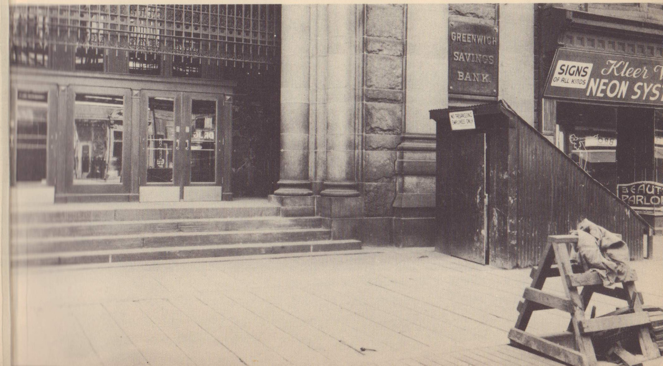
Here is a place (above) where the sidewalk decking is only a narrow bridge. Excavation work is going on where the rest of the sidewalk should be. The strange looking little outhouse in the picture below is actually the entrance to a flight of steps going down to the excavation itself. This is the way the workmen get down to their jobs.
