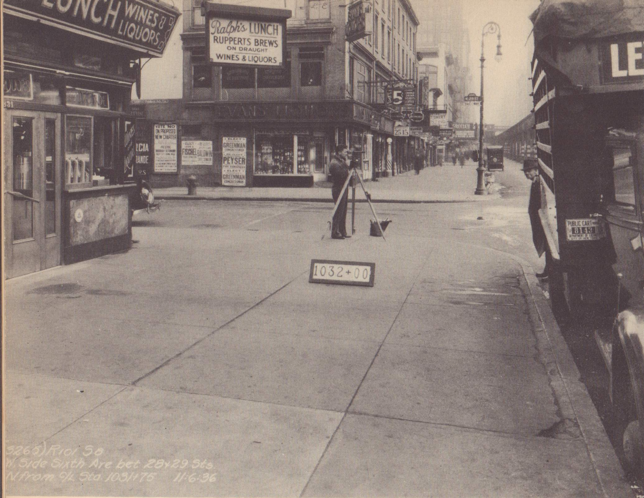
Here a surveyor is checking his base line with a transit. The board in front of him with the figures on it contains the number of the surveyor's "station" which he is checking.
