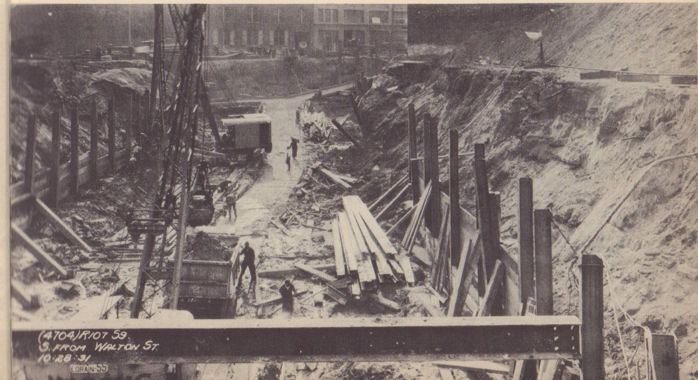
Excavation in open cut. No decking is needed. Above, a very wide street, with digging going on along half of it, without any temporary roadway. Below—Excavation across a vacant area.
