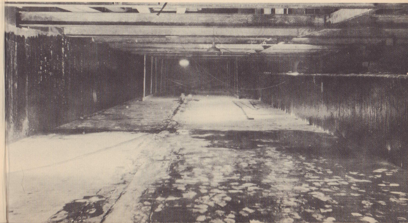
Here the waterproofing is shown. The photo above shows the brick-in-mastic being laid; and that below shows fabric waterproofing in place both on the floor and the walls of the subway.
