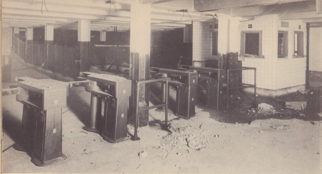
Station finish. A row of automatic turnstiles, operated by a nickel in the slot, is shown above, together with a specially built-in change booth, just beyond the turnstiles. That type of change booth is no longer used on the new subways. The one shown in the picture below is standard equipment nowadays.
