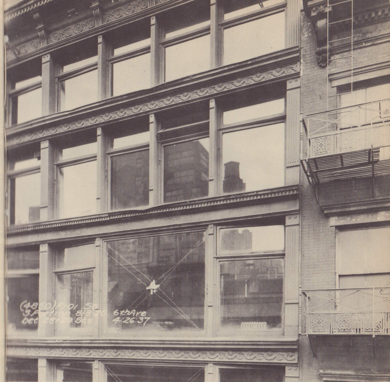
A window protector fastened on a big piece of plate glass. The engineers have figured out that the smaller windows in this building will not need protection, but that the big one might smash without it.
