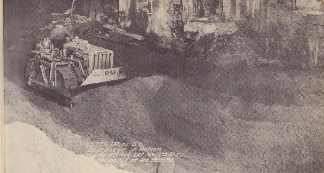
The bulldozer above is pushing the loose earth in toward the place where the power clamshell digger up on the sidewalk (see the picture below) can grab a mouthful of it in its jaws and lift it up.
