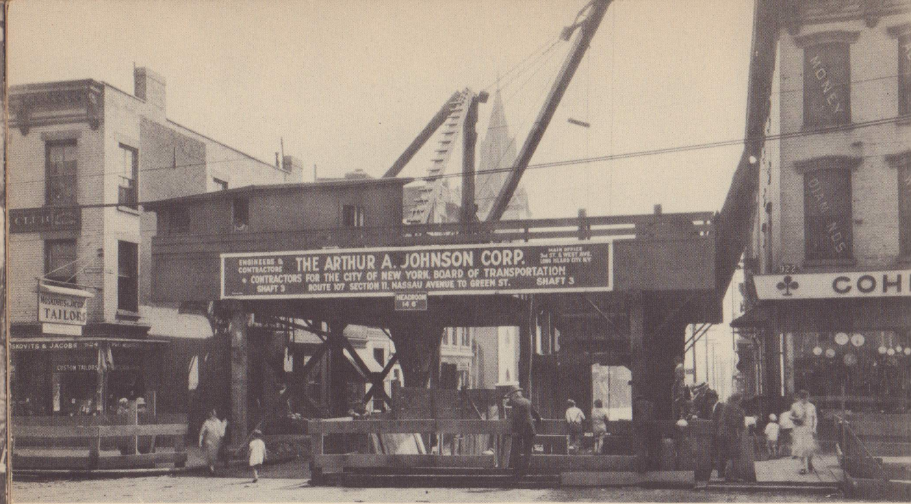
Another type of shaft (above) in which a "stationary crane" hoists material in buckets and dumps them into trucks. The queer contraption below is known as a "telpher"; it is a kind of shaft which moves along with the excavation as it proceeds! It is on log rollers, you will note. The telpher method is very rarely used, being cumbersome and awkward.
