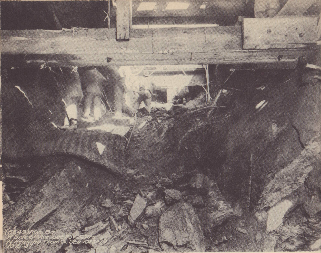
The blasting mat is in place, and the workers are scrambling out of the excavation before the blast is set off. Unfortunately, you cannot take a picture of a dynamite blast!
