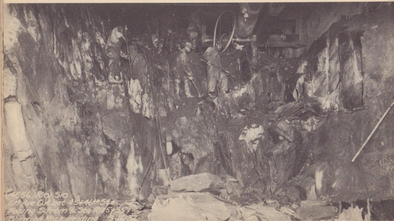
The drillers in the picture above are working with short drilling arms, and are putting down dynamite holes right up against the heading. The next blast may knock out several feet of the rock. Below, a blast has been set off, and the workmen are clearing up after it, pushing pieces of broken rock down to the bottom.
