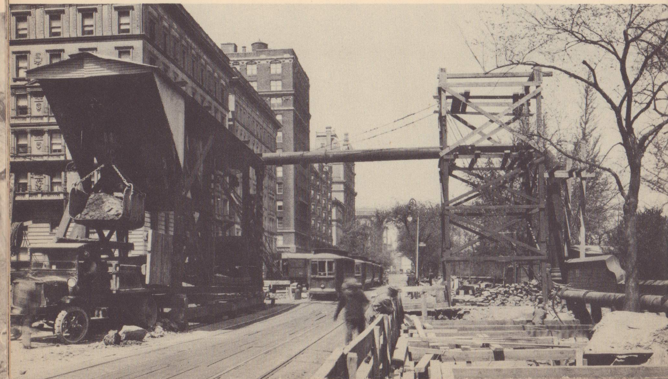
Another type of shaft (above) in which a "stationary crane" hoists material in buckets and dumps them into trucks. The queer contraption below is known as a "telpher"; it is a kind of shaft which moves along with the excavation as it proceeds! It is on log rollers, you will note. The telpher method is very rarely used, being cumbersome and awkward.
