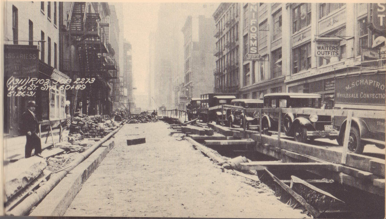
The construction contractor's last job on station platforms is putting in the reinforcing steel rods, and then covering them with a layer of concrete. Below—Backfilling under way. Pretty soon traffic will be running on the backfilled part of the road, while the other half, where it now is going, will be getting its load of earth and rocks.
