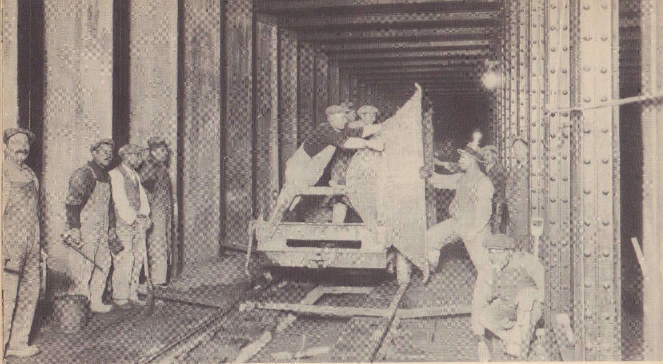
Concrete, mixed on the surface—frequently, but not always, in plants far away from the scene of construction, just as it was when the subway structure itself was being built—is dumped into the space between each tie and between the ties and the subway walls. Below—Another type of concrete cart.
