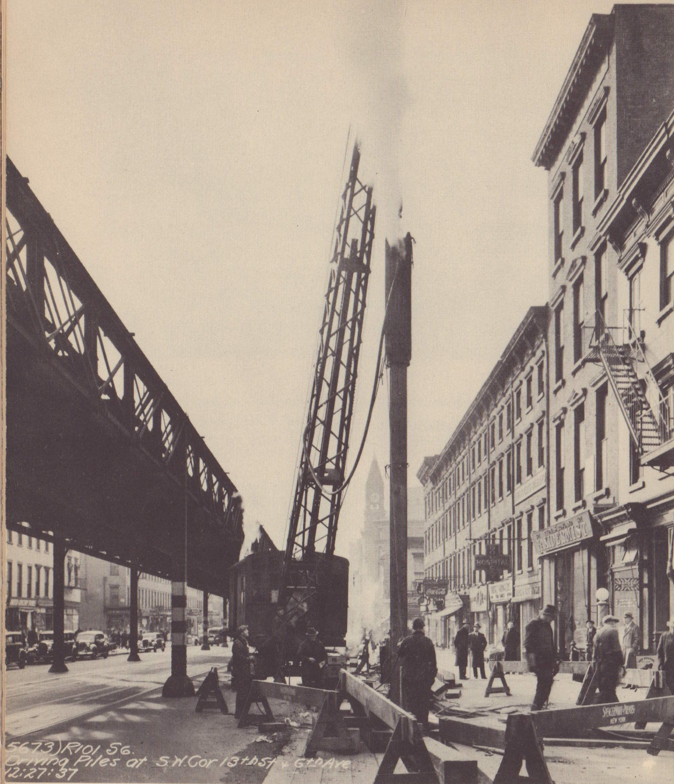
Driving the piles on which the decking will eventually rest.
