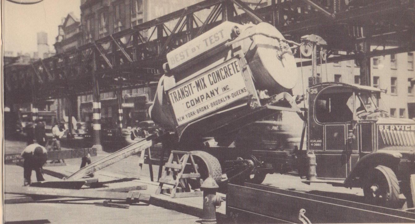
Here is the way concrete arrives at a modern subway construction job. No more do you find unsightly piles of sand, cement and crushed rock all along the street, waiting to be mixed into concrete. Below is the other end of the funnel into which the concrete is poured. This is the end it comes out of. (Top photo, courtesy of Spencer, White and Prentis.)
